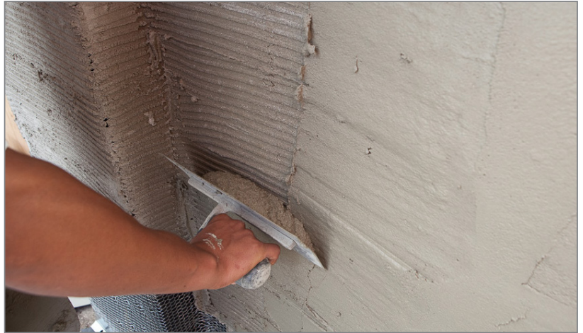
Application of proprietary, preblended, shrinkage compensated basecoat
